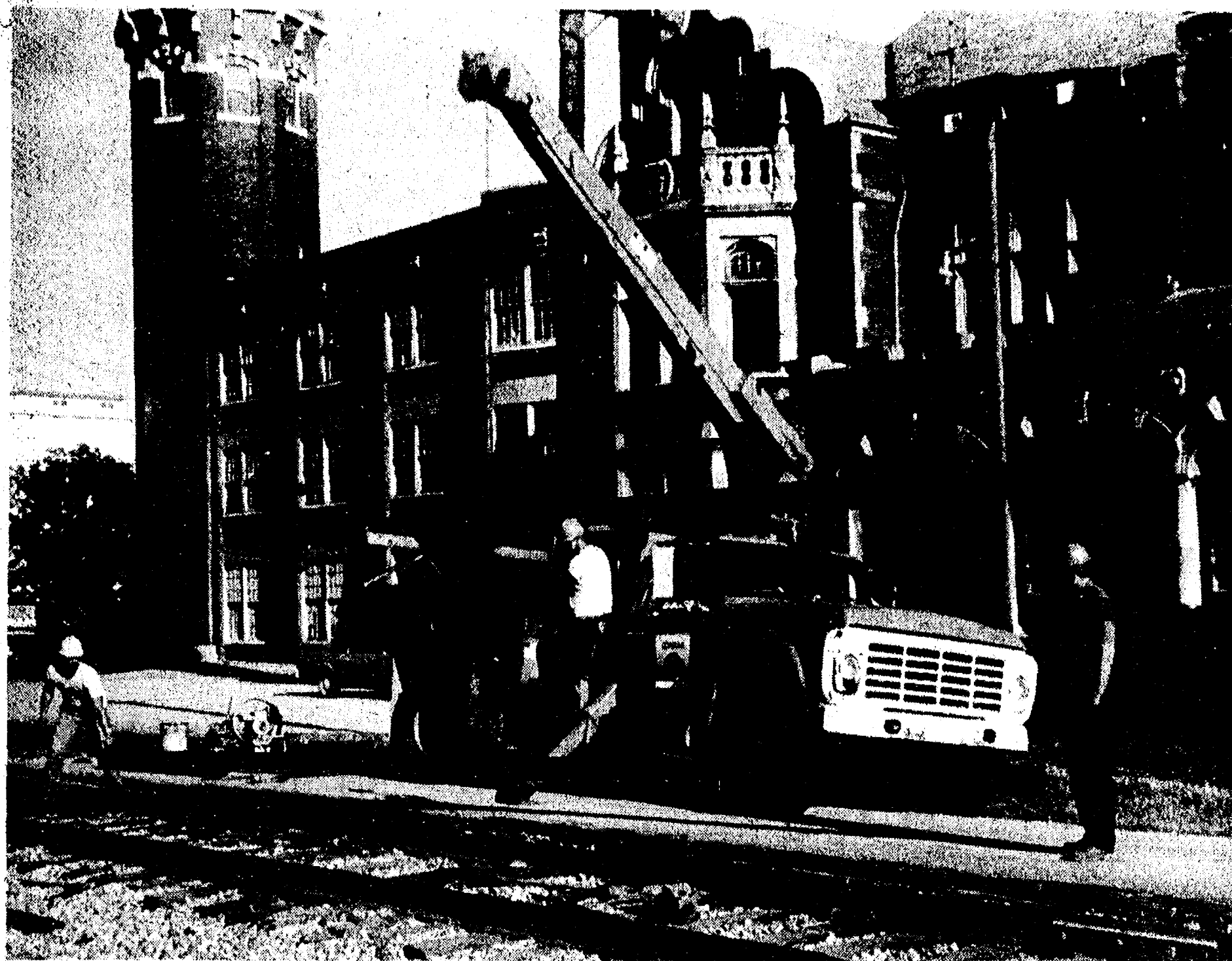
RAILS REPLACED: Sections of damaged rail were replaced along the Conrail tracks through Chelsea last week. The pieces requiring replacement are located by a sophisticated machine which detects differences in sound waves given off by good and bad rails.
