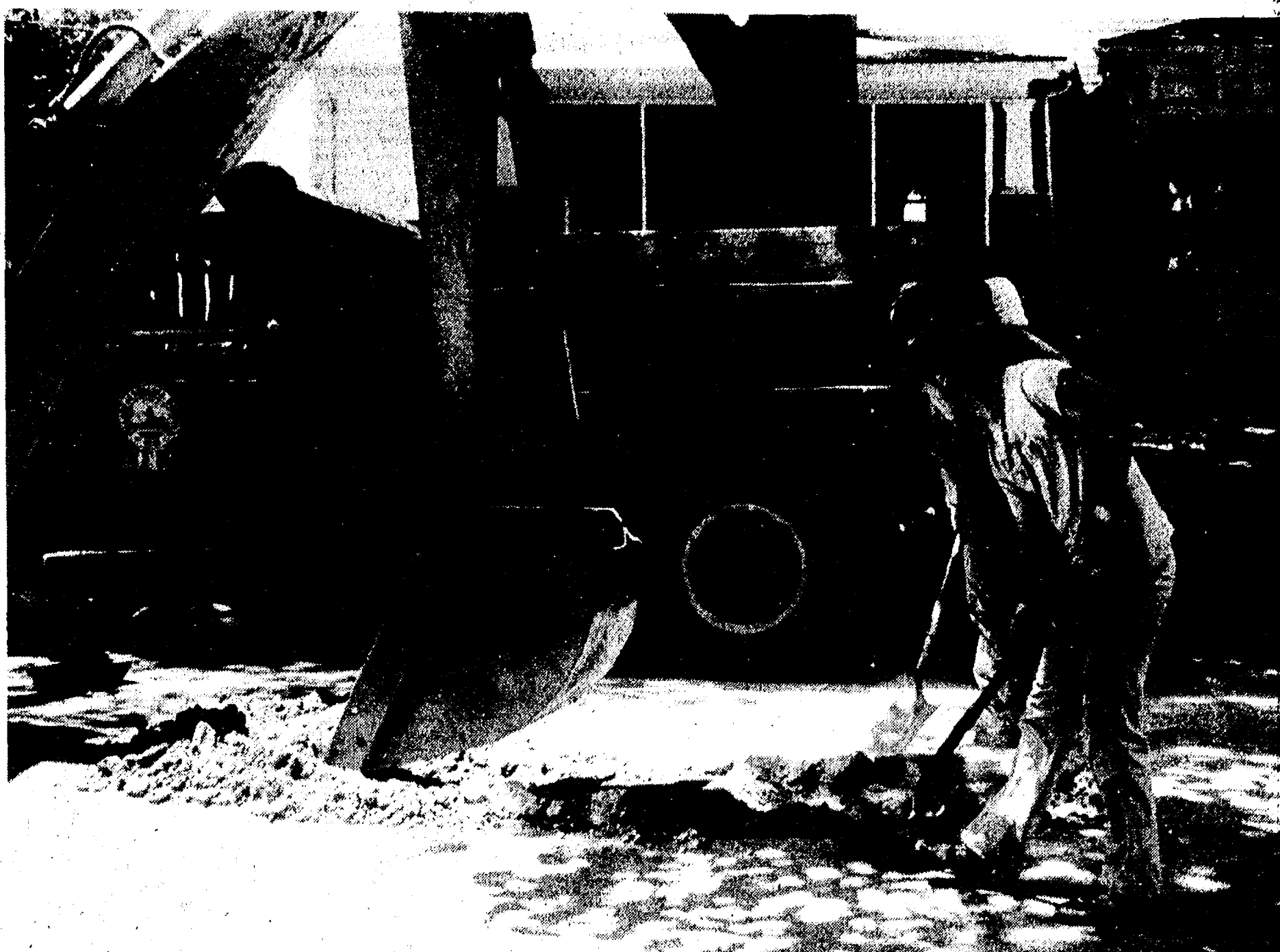
SUMMER IS THE TIME to fix streets, and village crews are busy patching holes and making other repairs. Part-time workers David Wojcicki and Dan Pennington (rear) were shovelling out a hole for hot-patch asphalt when this picture was taken on East St. last week.
